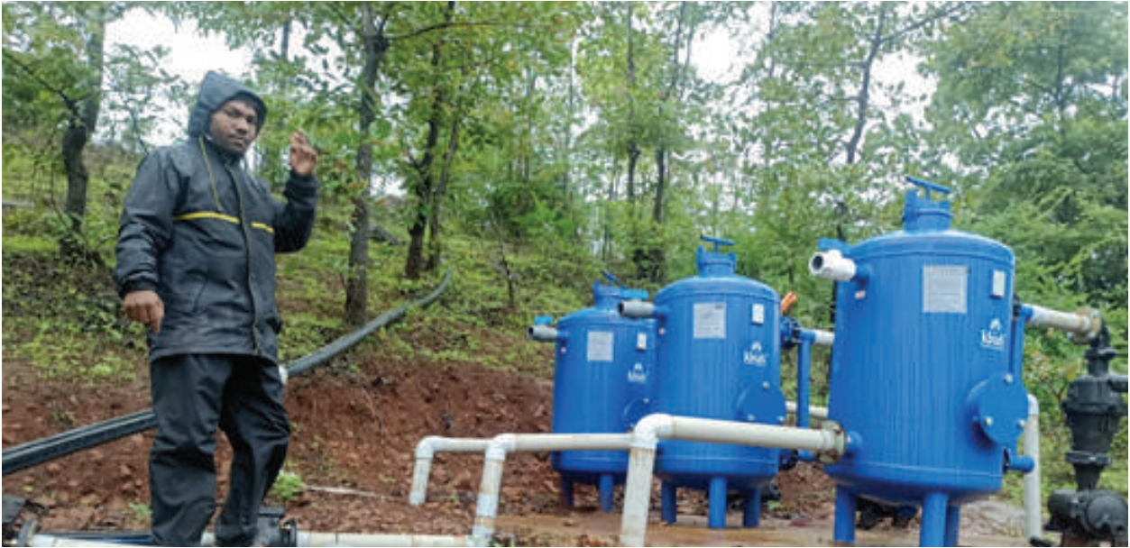
Observing the solar project in village
